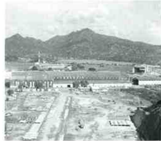
PT Cilegon Fabricators (INDONESIA) Products & services: Boilers, steel structures, container cranes and pressure vessels Certificates: ISO 9001 and ASME (S, U, PP)
